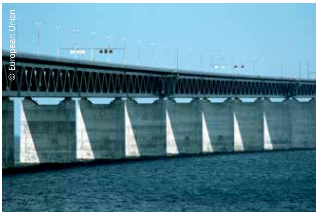
The Øresund bridge is the longest combined road and rail bridge in Europe.
